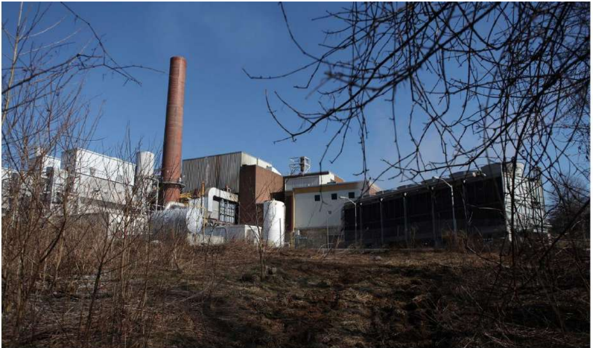
The Harrisburg Incinerator on South 19th Street. ((AP Photo/Carolyn Kaster))
